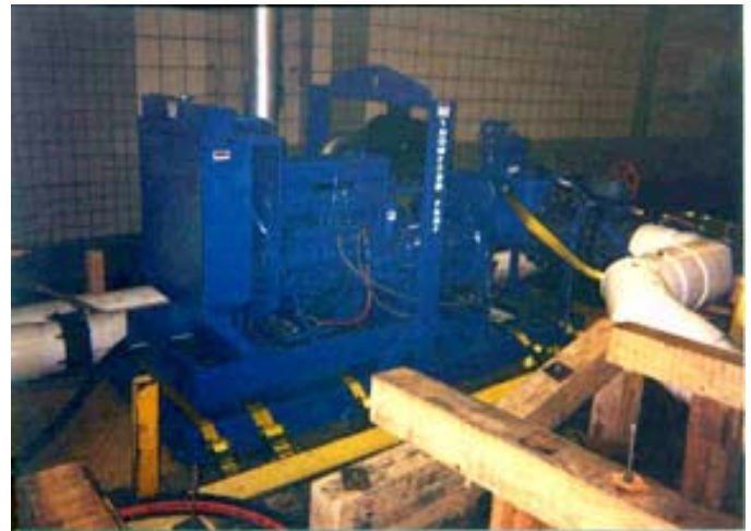
Pumps and piping are set up to begin the dewatering process.
