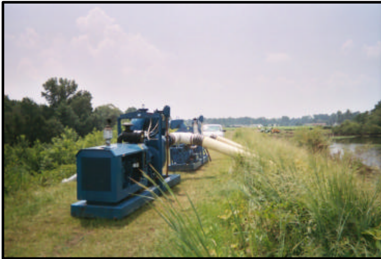
Two Thompson Pump Vacuum-Assisted Dry Prime Trash Pumps are installed on the earthen dam in order to lower the water level of Bear Creek Lake.
