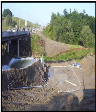
The wellpoint system is installed adjacent to a overpass.
