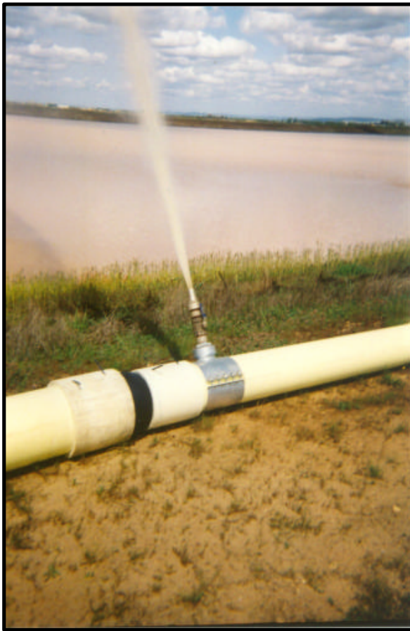
Fifteen one-inch nozzles were installed along the discharge pipe and expelled the water 80-feet into the air, causing most of the discharged water to evaporate into the air.
