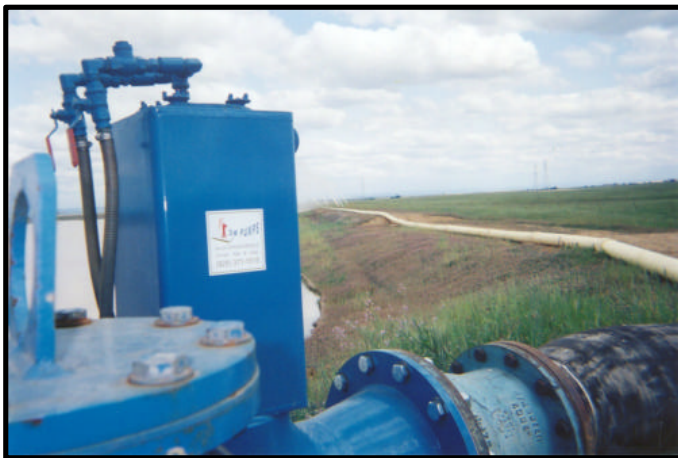
The system consisted of 1,800-feet of 12-inch discharge pipe.
