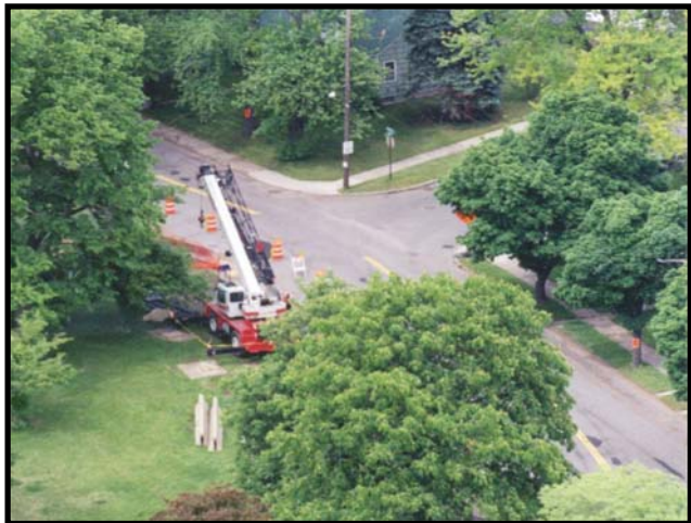
ITT Flygt submersible pumps are lowered into the manhole.
