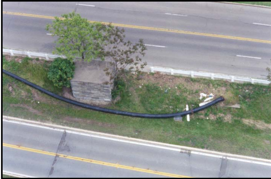
The bypassed sewage re-enters the main line.
