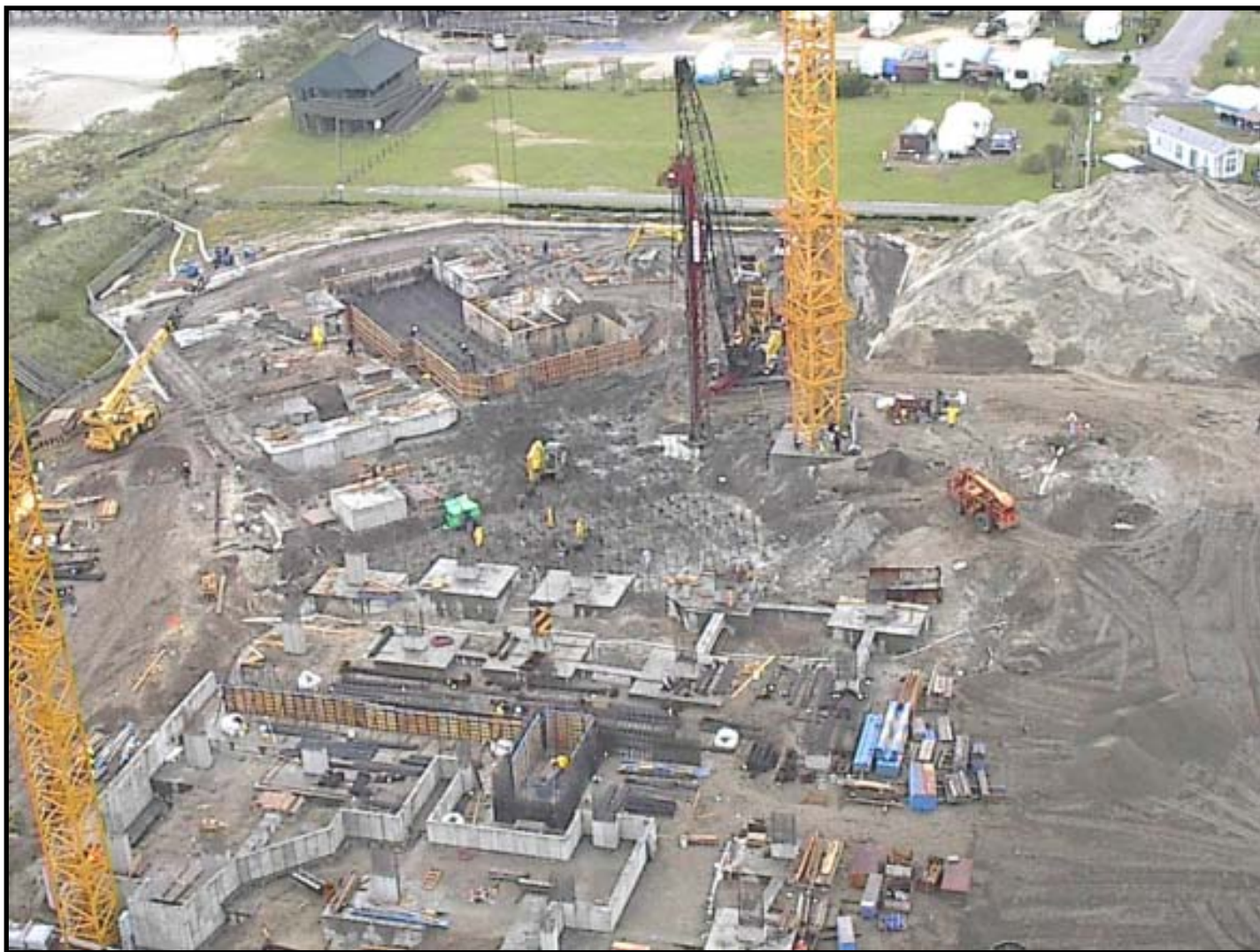
An overview of the entire construction site.
