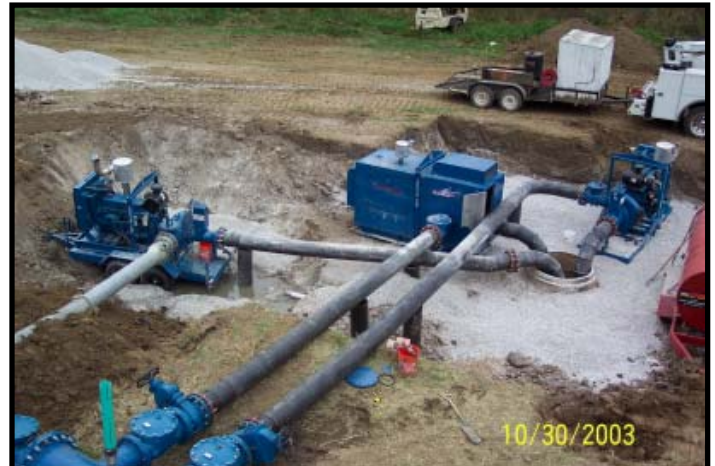
Three Thompson 12-inch High Pressure Solids Handling Pumps were installed to bypass the section of the interceptor that was in need of repair. Each of the pump's discharge lines fed into a single common manifold.
