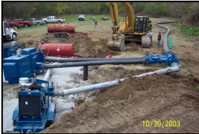
Three Thompson 12-inch High Pressure Solids Handling Pumps were installed to bypass the section of the interceptor that was in need of repair. Each of the pump's discharge lines fed into a single common manifold.
