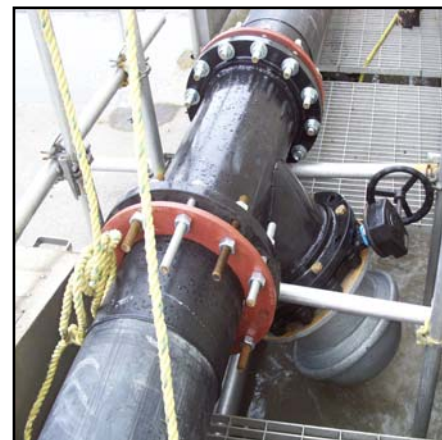
Two of the discharge points for the sewage from the manhole opening. Check valves and gate valves were used to regulate the flow, and to have the ability to open or close sections of the discharge system.
