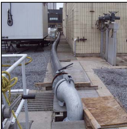
Two of the discharge points for the sewage from the manhole opening. Check valves and gate valves were used to regulate the flow, and to have the ability to open or close sections of the discharge system.
