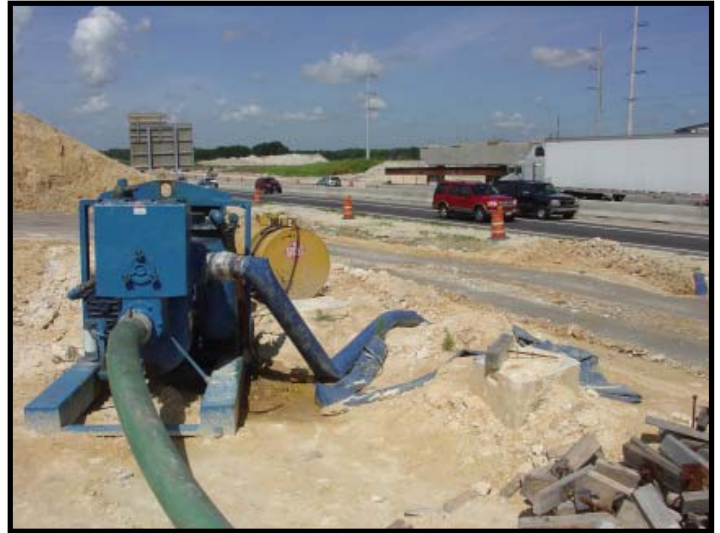
A Thompson Pump 8-inch Vacuum Wellpoint Pump dewatering a rim ditch to assist with the construction of a new bridge that will cross over the busy interstate.
