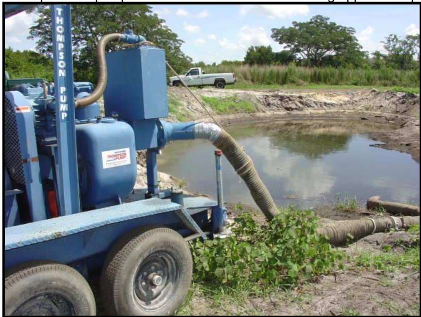
Another Thompson 8-inch Vacuum Wellpoint Pump dewatering a pond that will be further excavated and a rubber lining will be installed to protection the pond floor.
