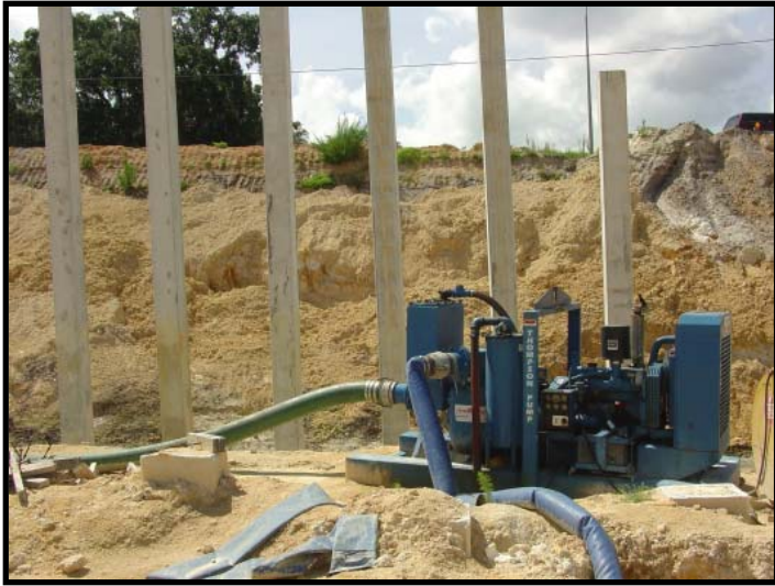
A Thompson Pump 8-inch Vacuum Wellpoint Pump dewatering a rim ditch to assist with the construction of a new bridge that will cross over the busy interstate.
