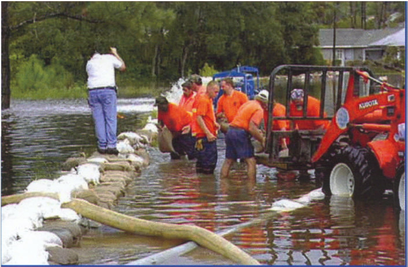
A picture from the front page of the Daytona Beach News-Journal. A work crew builds a makeshift sandbag wall to stem the flow of water from a nearby lake, using Thompson Pump trash pumps.
