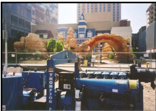
Thompson Pump's 12-inch Rotary Wellpoint Pump dewatering the Bally's/Caesars Parking Garage
