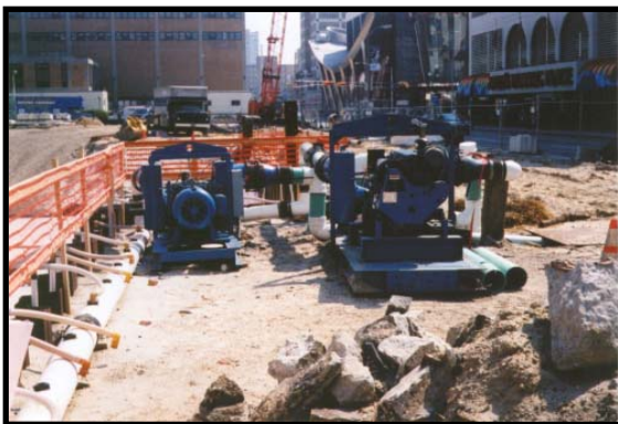
Thompson's 12-inch Rotary Wellpoint Pumps on the Bally's/Caesars Parking Garage project.
