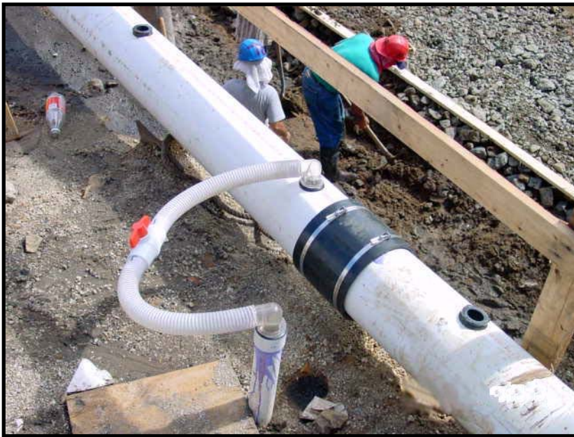
Crews began excavating as the wellpoint system was in operation.
