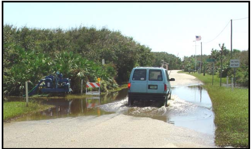
Above and Below: A delivery van wades through flooding on this main access road in Ponce Inlet, FL after Hurricane Jeanne. Ponce Inlet is the last town in Volusia County on the north peninsula that separates the Atlantic Ocean from the Intercoastal Waterway. Thompson Pump's 4" Dry Prime Vacuum Assisted Trash Pump works on removing the water from the area, which included a local water treatment plant.
